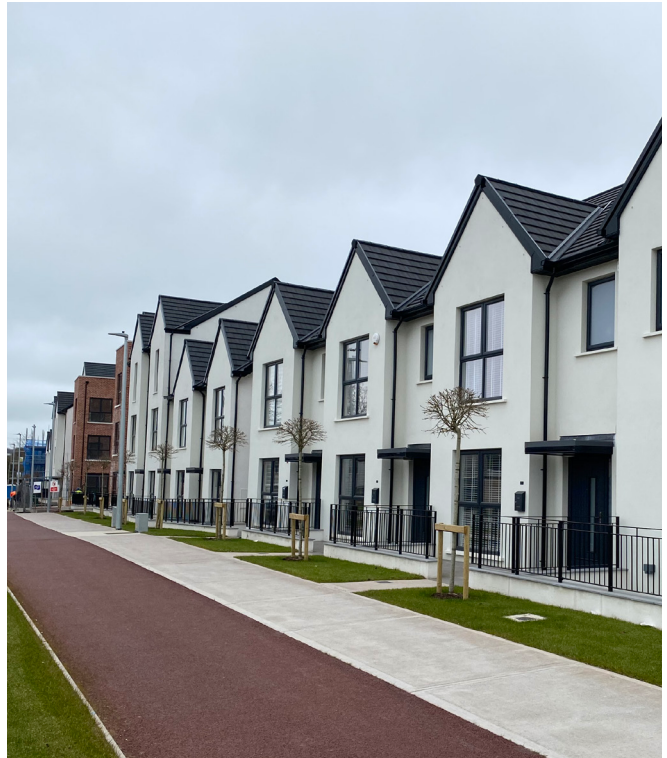
Figure 8: New Residential Development
