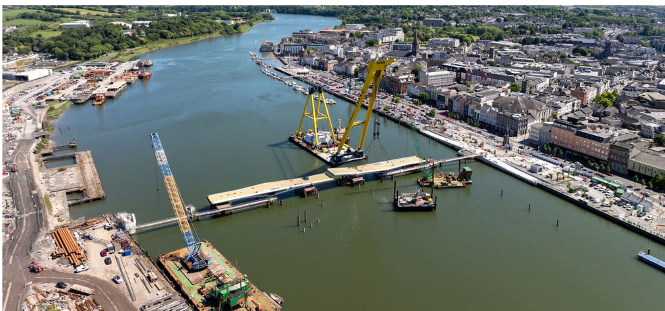
Figure 2: Installation of Sustainable Transport Bridge to North Quays (Source: Waterford City and County Council)
