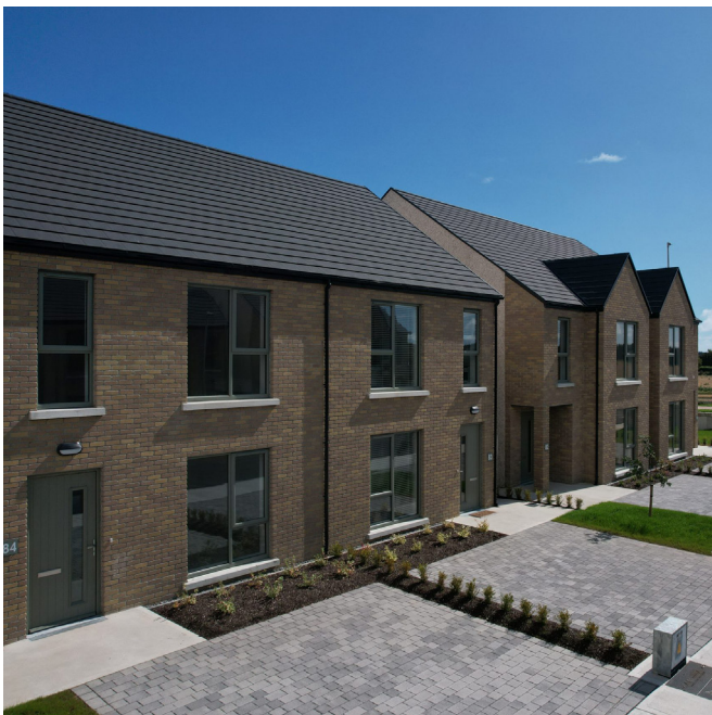
Figure 3: Summerfields Housing Development (Source: Whitebox)
